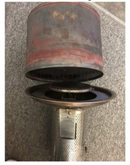
2. Remove four screws around emitter grid.
